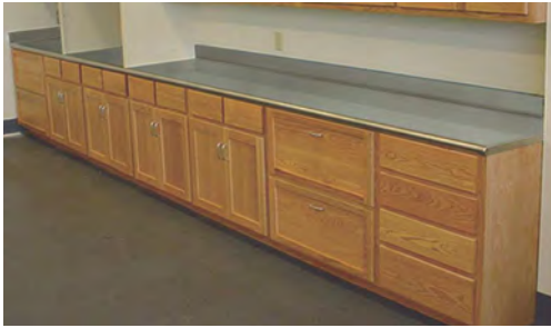
stainless steel countertops fabricated to drawings indicating backsplash height, raised edge and field condition requirements
